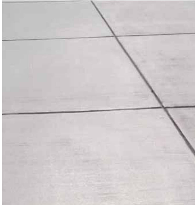
Plain Concrete Paving Broom finish
